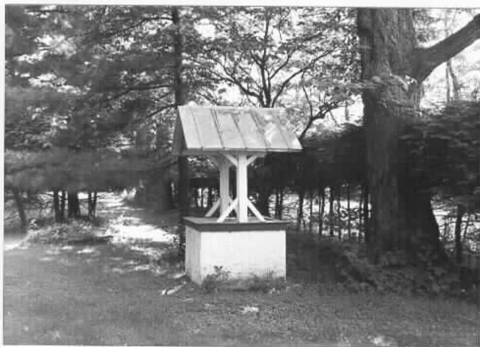
5 Well house, viewed from north
