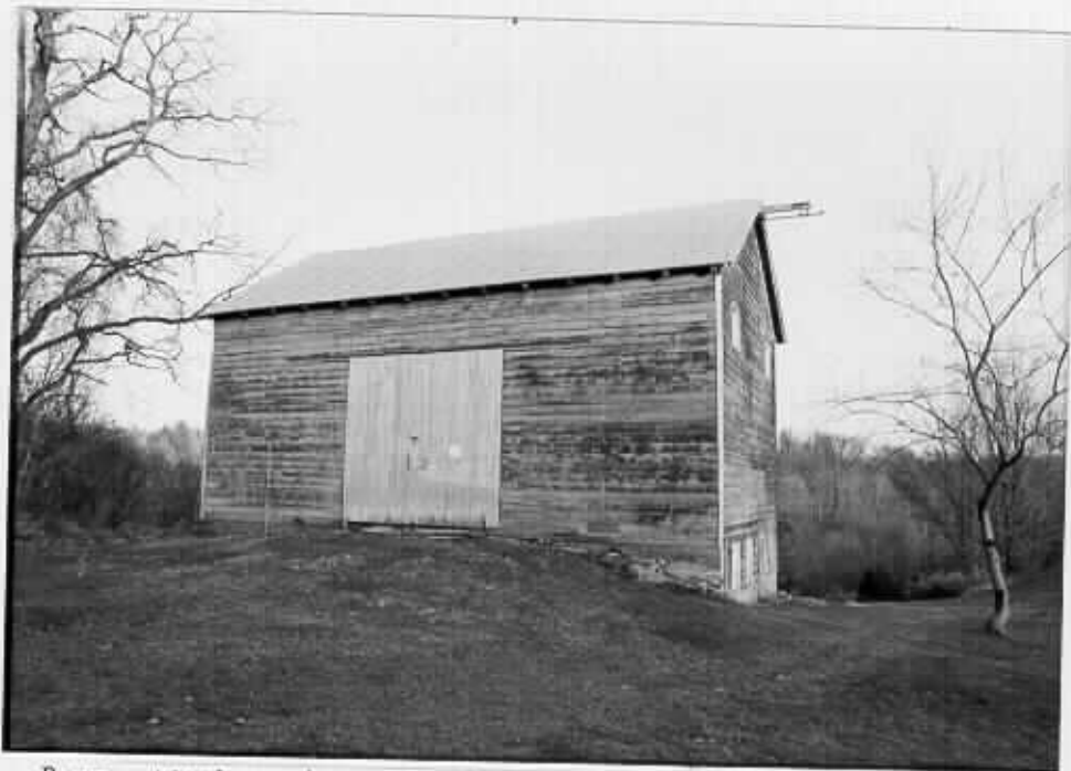
6 Barn, west and south elevations, viewed from west
