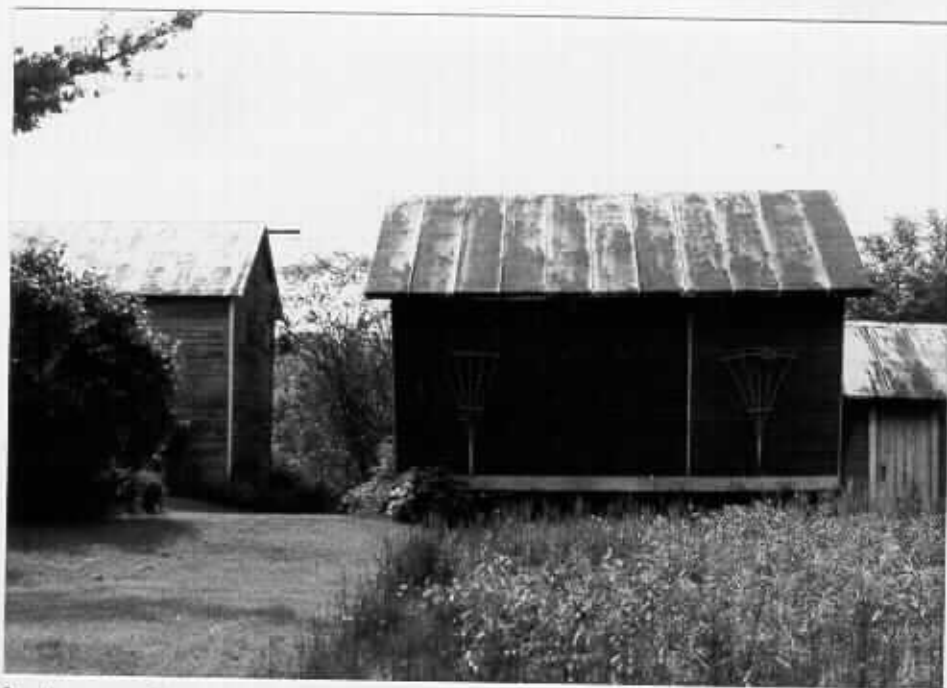
7. Corn crib and shed, west elevation
