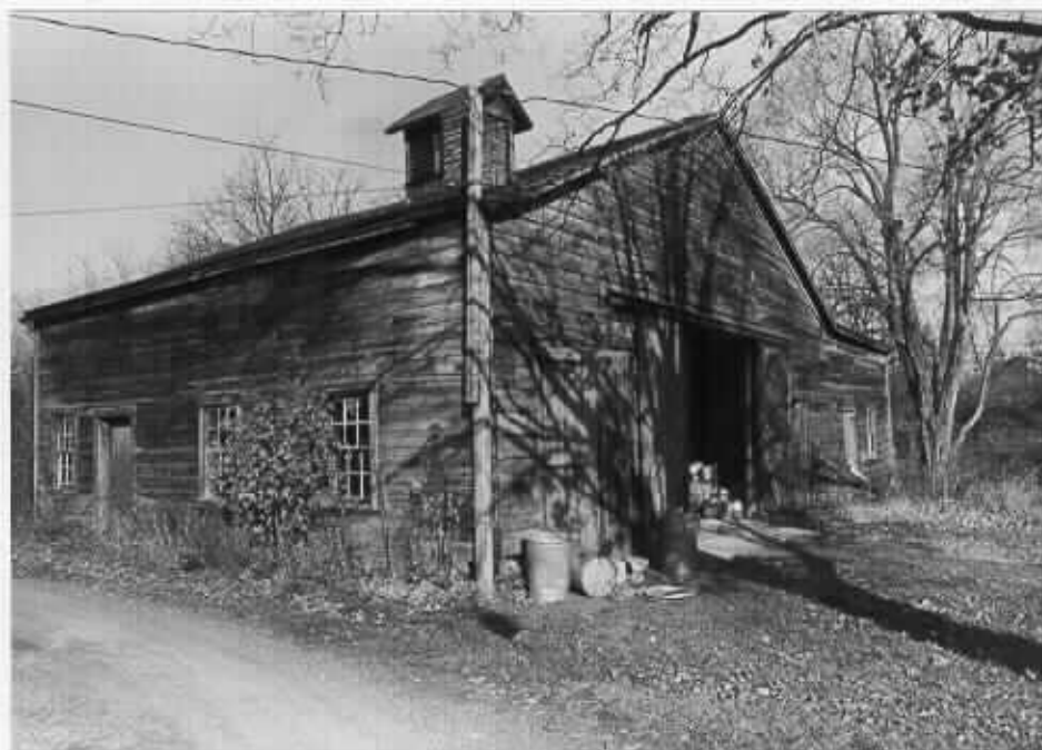
16 Wagon shed, south and west elevations
