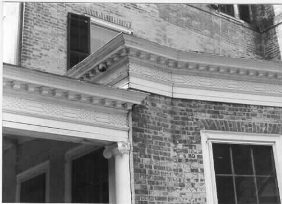
8 Manor house, porch and cornice details
