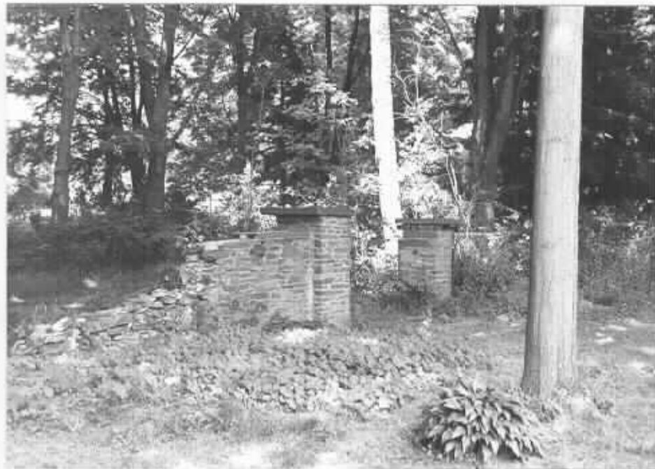
9. Remains of gates, northwest of manor house marking former access to tenant house
