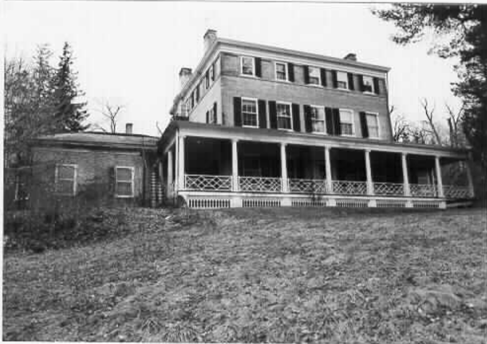
3. South facade and west elevation with one-story library wing
