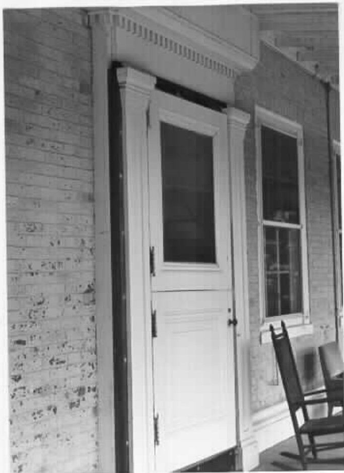
6. Main block, south facade Center entrance
