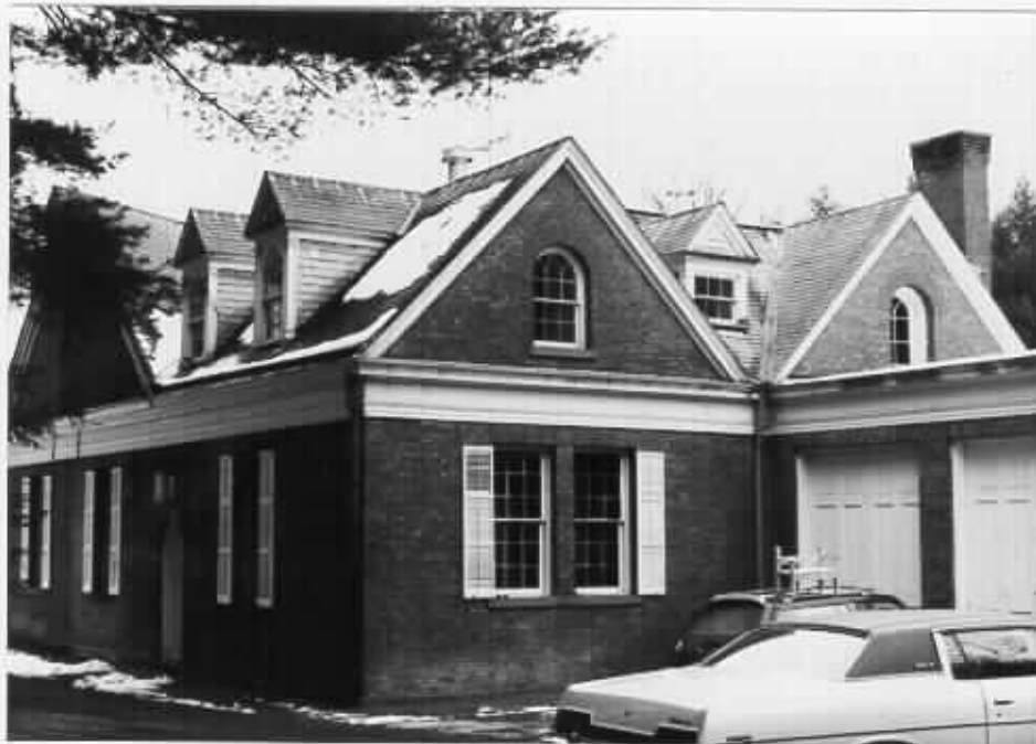
18. West facade and south elevation
