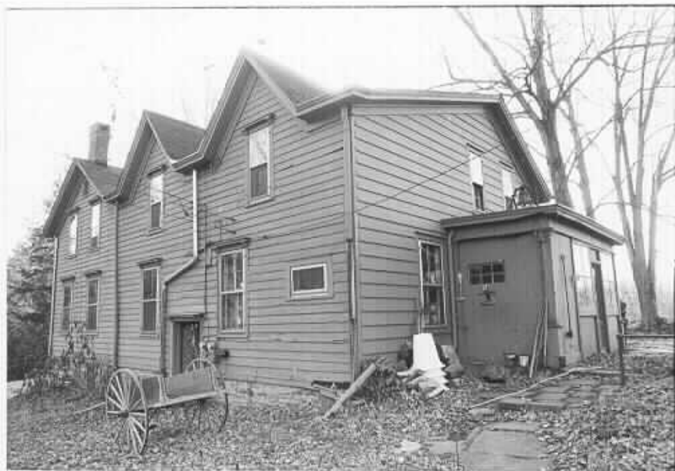
15. East and north elevations
