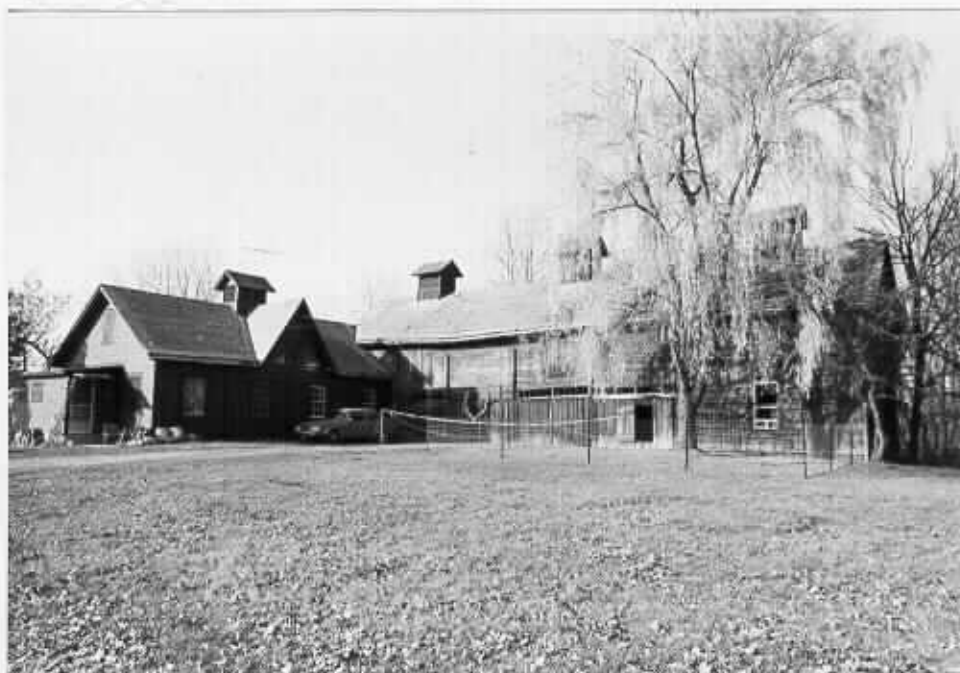
17. Barn complex, south and east elevations
