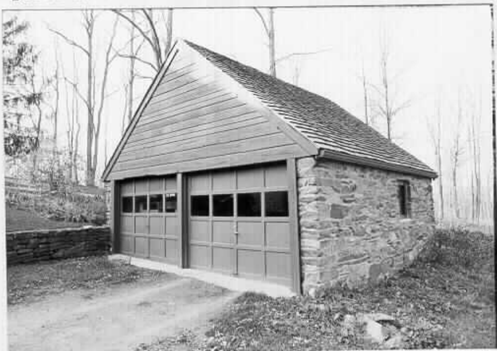
5. Garage, south and east elevations
